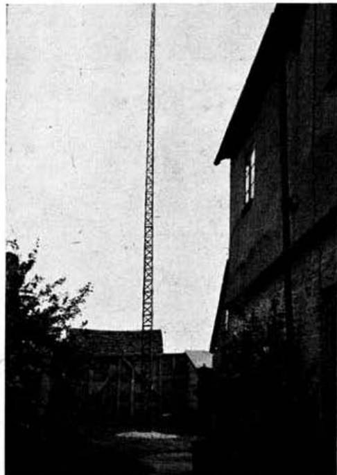
Wooden Aerial Mast constructed by Mr. Long, GSLO.
